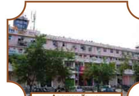
Agarsen Tower Residential Project 13, Central Spine, Vidyadhar Nagar Jaipur 27 माह में पज़ेशन
