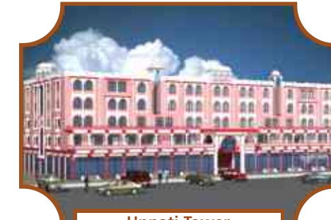
Unnati Tower Commercial Project Central Spine Vidyadhar Nagar, Jaipur 20 माह में पज़ेशन
